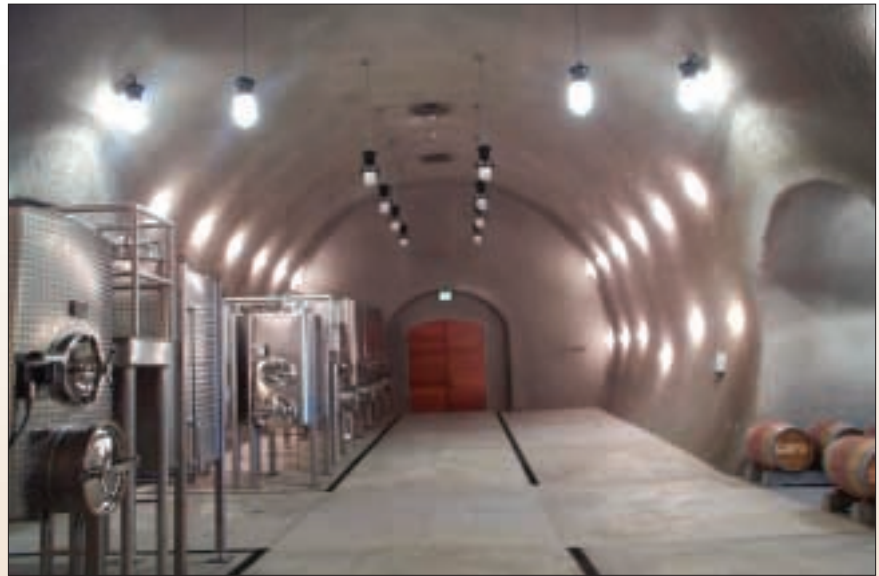
The storage of wine underground offers the benefits of energy efficiency and optimum use of limited land area.
